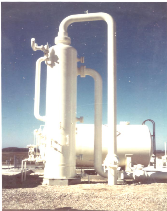
Fig. 1B—A field installation for a high G-force vertical recycling separator is illustrated.
